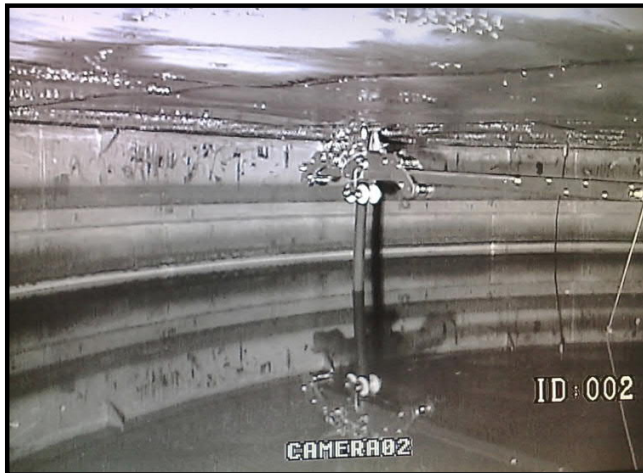
Retrieval - view inside the tank - pumping arm (180° rotated), remotely controlled from control room
