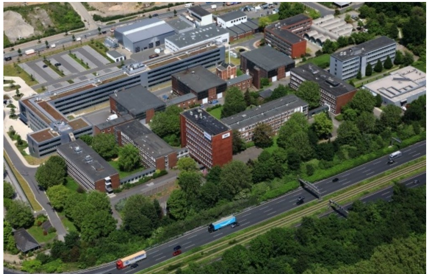
Figure 14. DMT building in Essen Germany.
